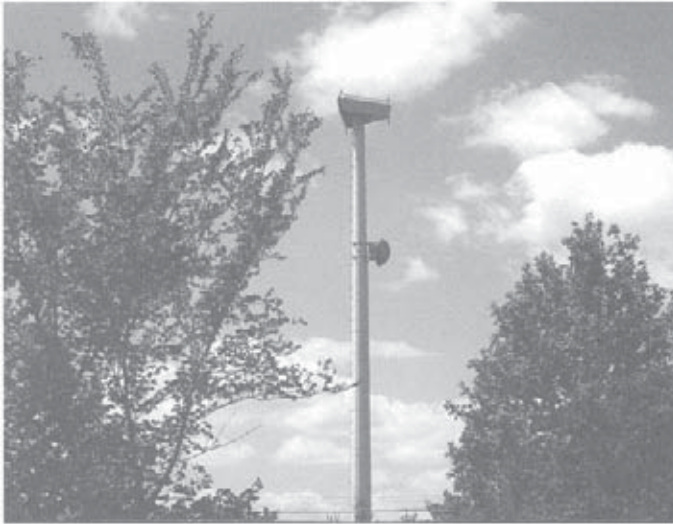
Fig. 6. A typical cellular tower.
